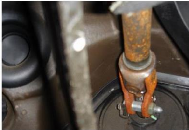
转向柱及万向节缝隙腐蚀
